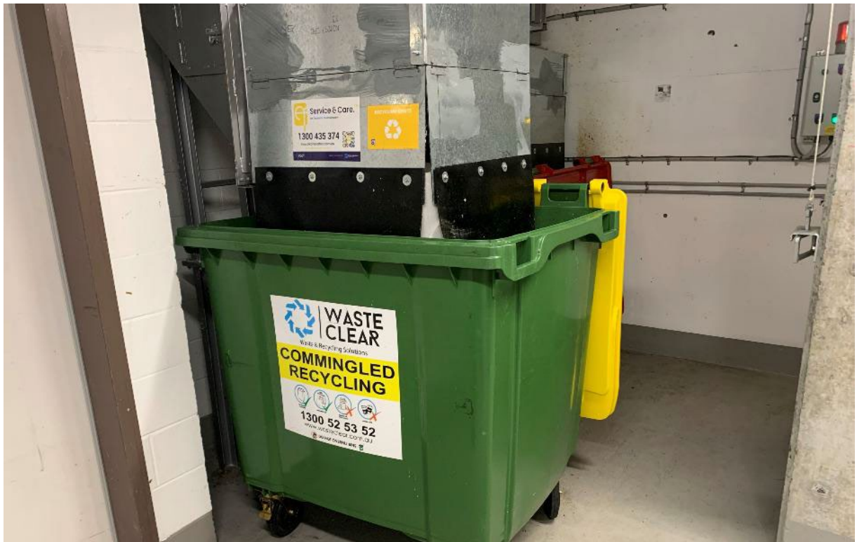
Waste chute connected to waste storage area.
